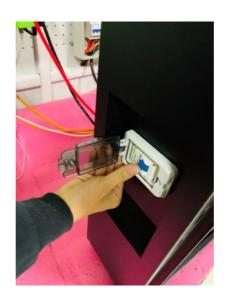
Step 8: Power on DC breaker between battery and inverter.
