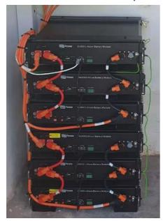
Because 1 pair of power cable Max. continuous current is 120A,if the current is too high on one cable,it will cause the socket and plug temperature become too high,affect the battery performance.
