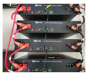
Step 7:Switch on DC breaker between the battery system and inverter
