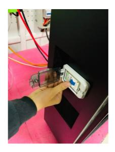
Step 8: Power on DC breaker between battery and inverter.
